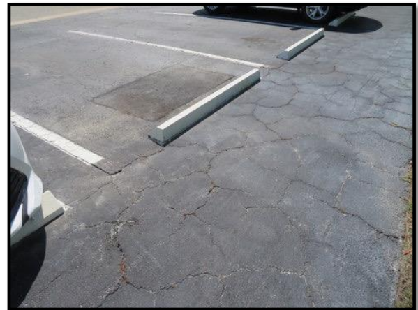
Figure 2 - Significant Cracks
