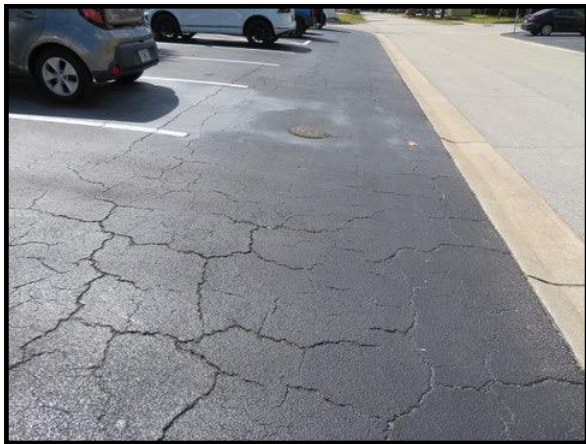
Figure 1 – Significant Cracks
