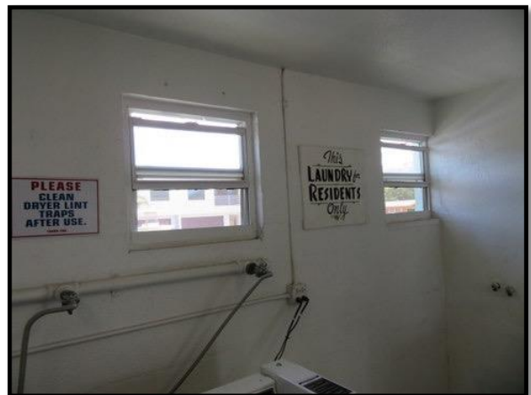
Figure 2 – Laundry Room Windows
