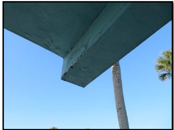
Figure 2 – Beam Crack
