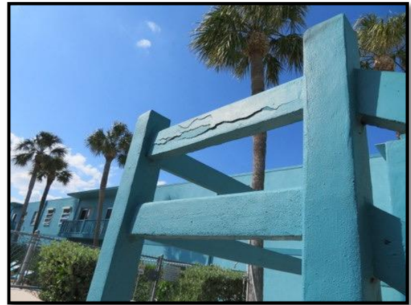
Figure 2 – Railing Cracks
