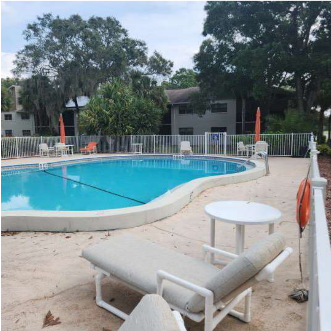
5 5-POOL Date Taken: 10/13/2023 Taken By: Michael Weekly THE OAKS OF COUNTRY CLUB CONDOMINIUM ASSOCIATION, INC. 1600 WOODLAND RD. ROCKLEDGE, FL 32955
