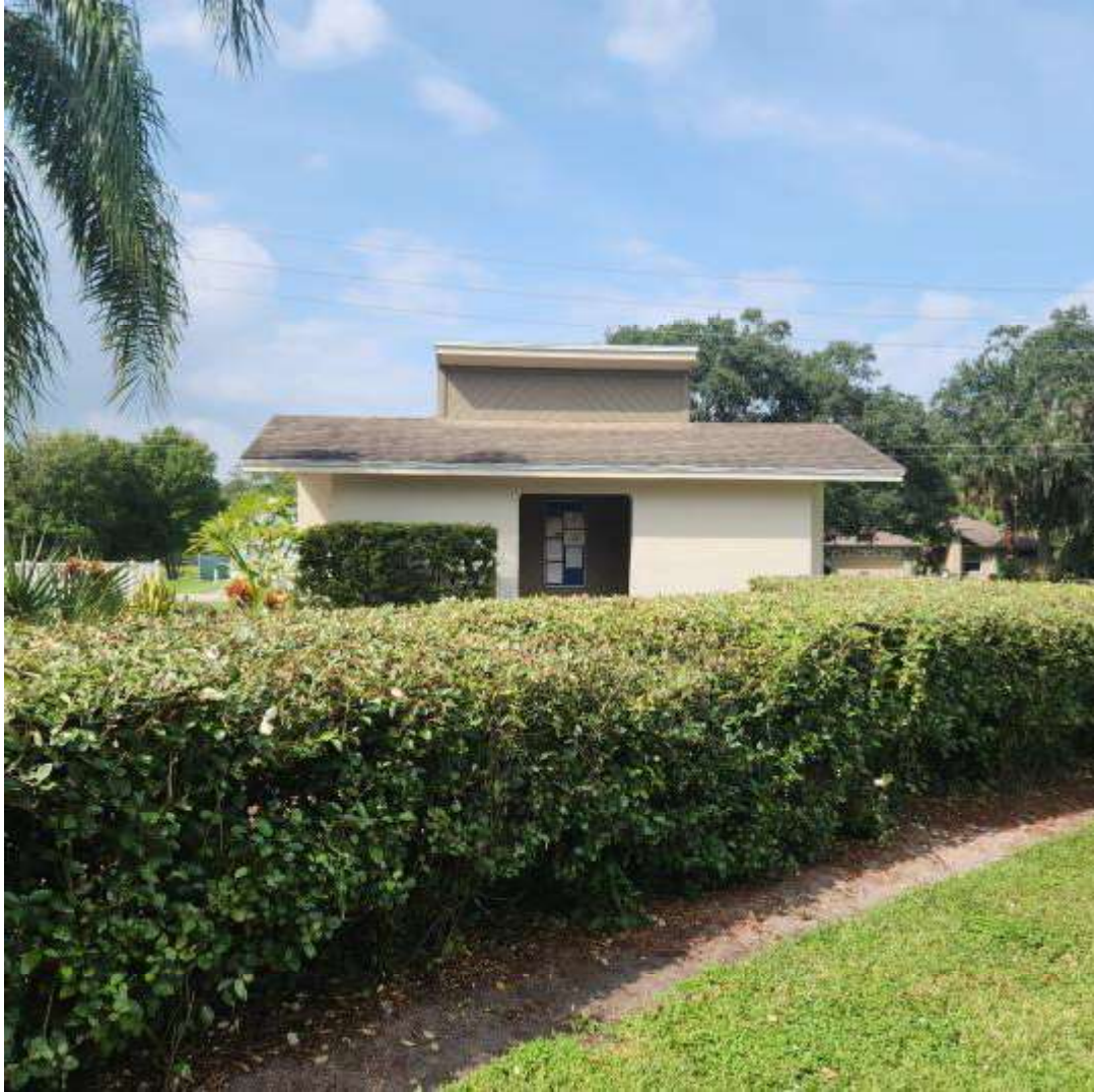
2 2-POOL RESTROOM Date Taken: 10/13/2023 Taken By: Michael Weekly THE OAKS OF COUNTRY CLUB CONDOMINIUM ASSOCIATION, INC. 1600 WOODLAND RD. ROCKLEDGE, FL 32955
