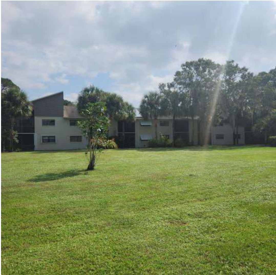
10 10-REAR 4101-4206 Date Taken: 10/13/2023 Taken By: Michael Weekly THE OAKS OF COUNTRY CLUB CONDOMINIUM ASSOCIATION, INC. 1600 WOODLAND RD. ROCKLEDGE, FL 32955
