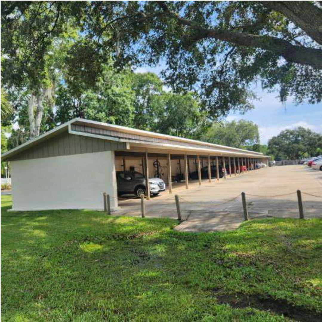
17 17-CARPORT Date Taken: 10/13/2023 Taken By: Michael Weekly
