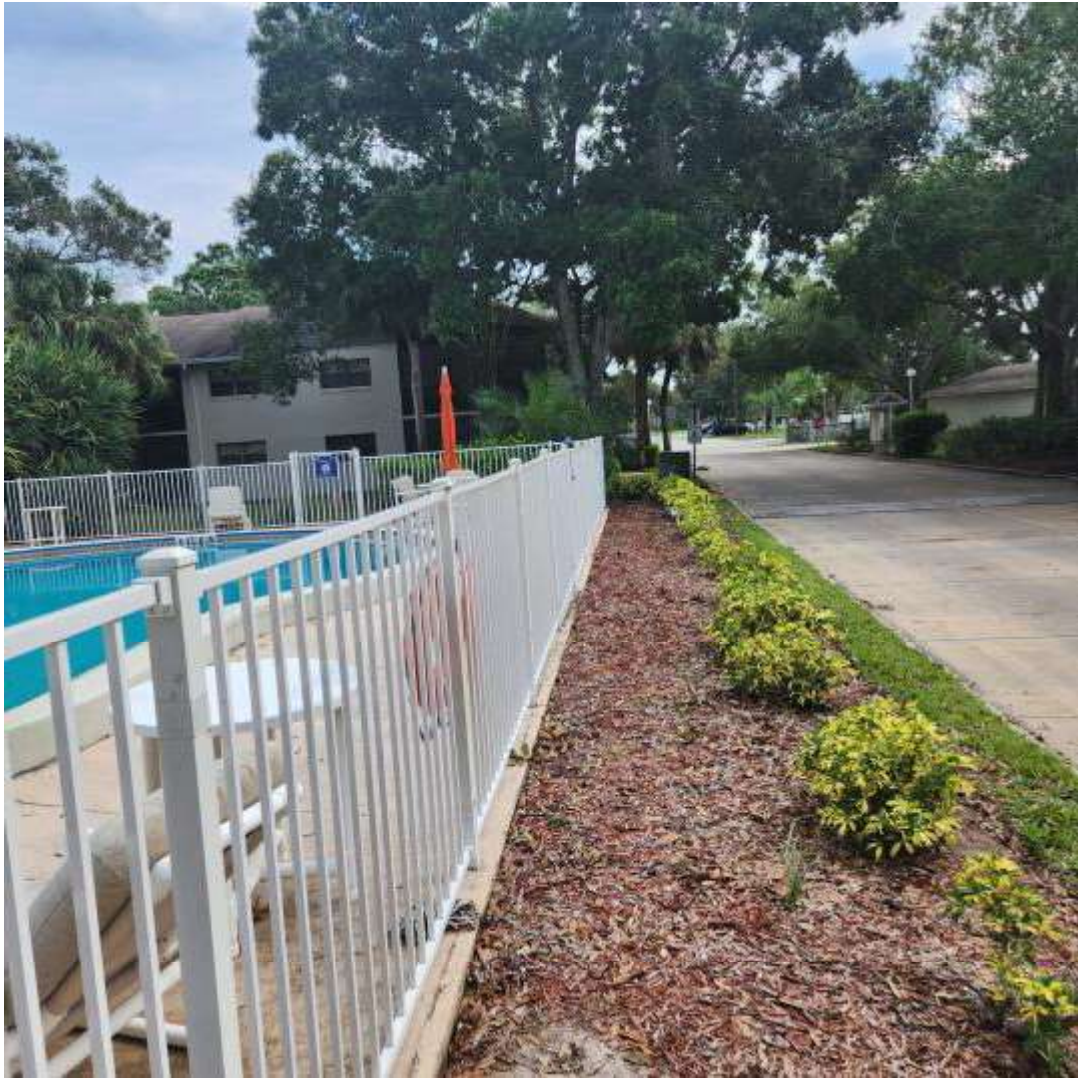
7 7-POOL FENCE Date Taken: 10/13/2023 Taken By: Michael Weekly THE OAKS OF COUNTRY CLUB CONDOMINIUM ASSOCIATION, INC. 1600 WOODLAND RD. ROCKLEDGE, FL 32955
