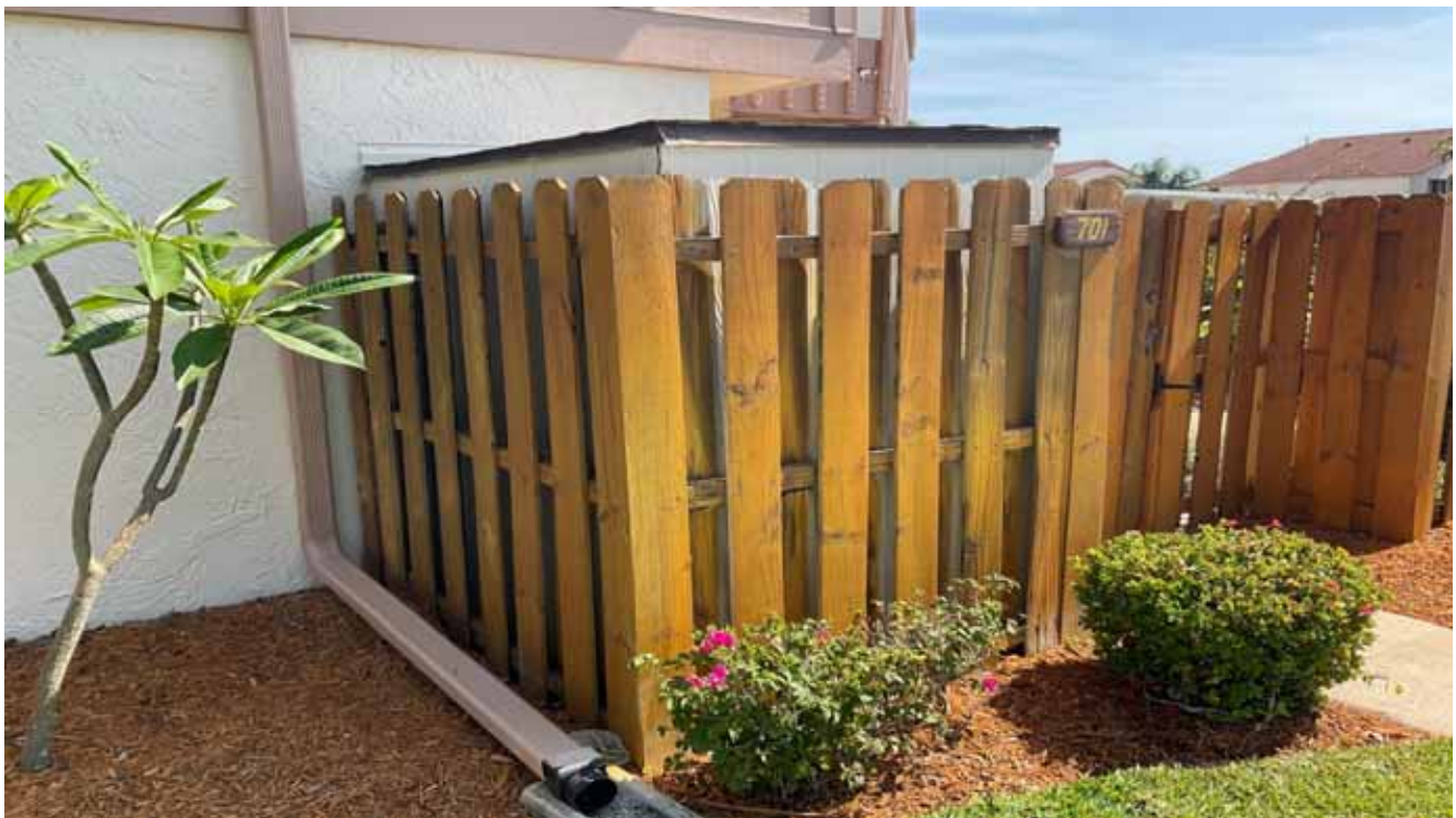
Shed at Villa's - Typical
