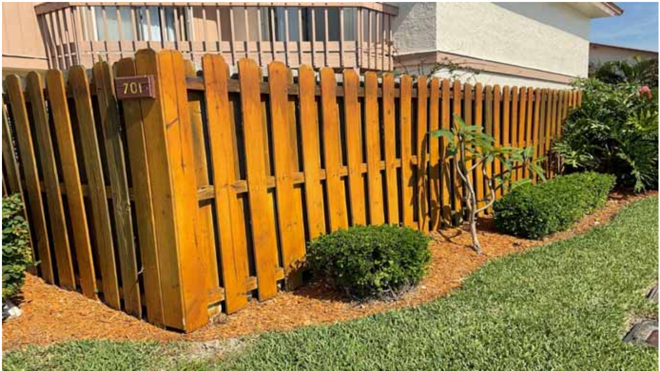
Fence at Villa's - Typical
