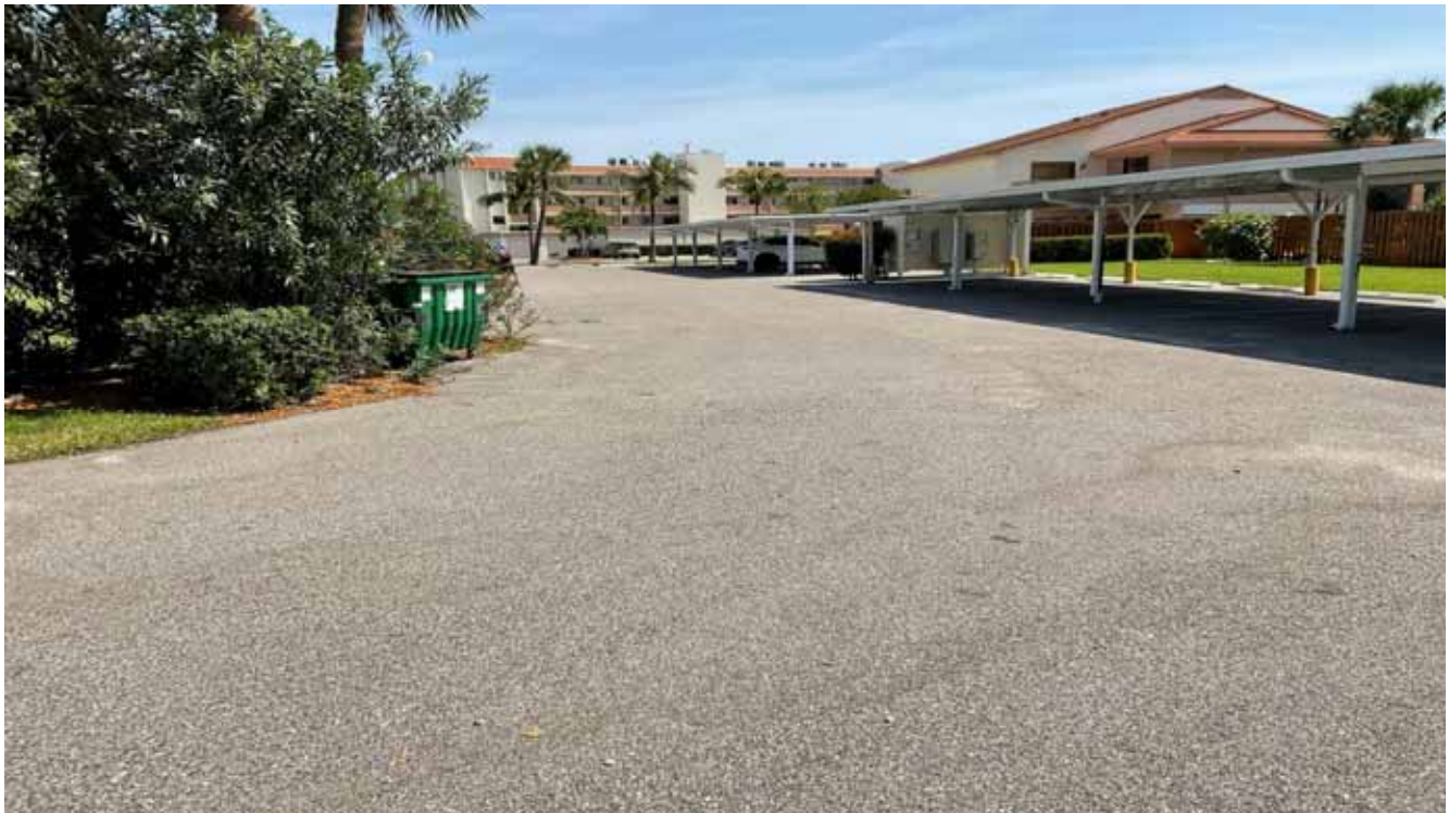
Parking Lot - Section III
