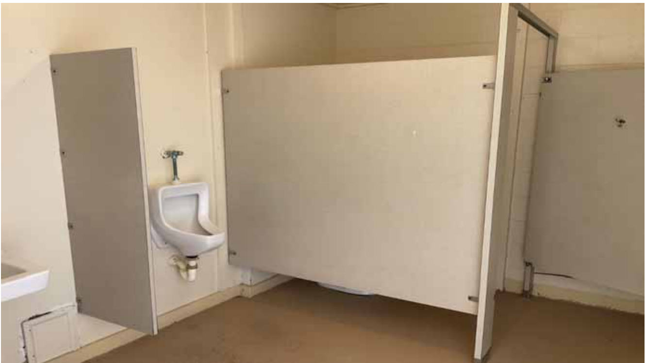
Pool Restroom - Midrise
