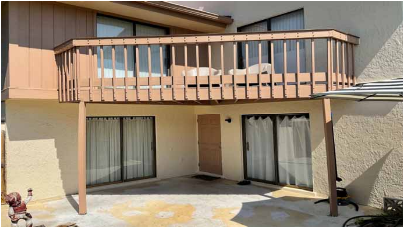
Balcony Deck at Villa's - Typical
