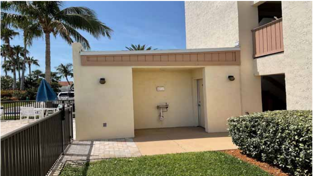
Pool Restroom - Midrise
