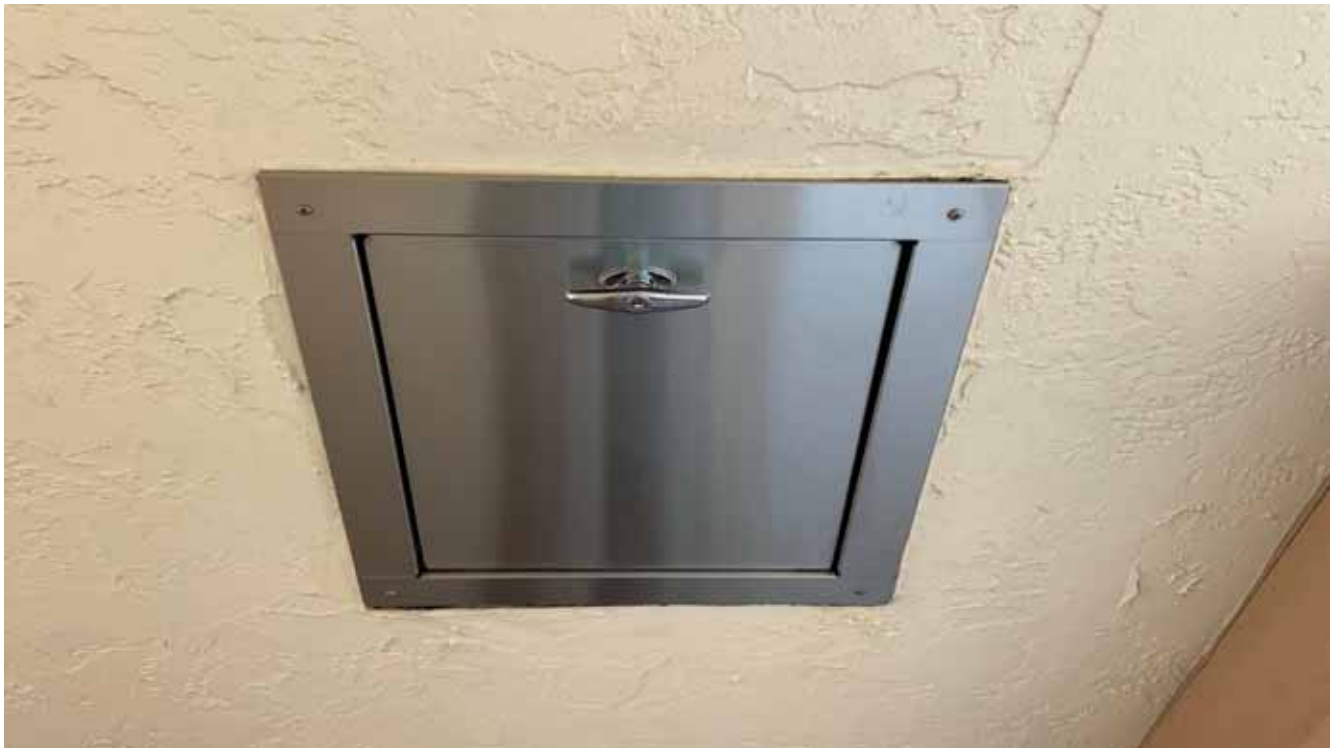
2400 Bldg - Trash Chute
