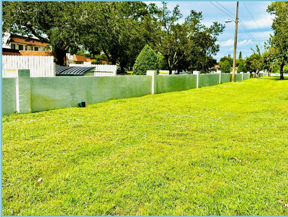
WEST PERIMETER WALL
