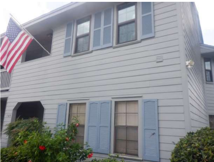
Openings not protected
