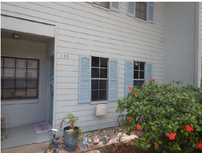
Openings not protected
