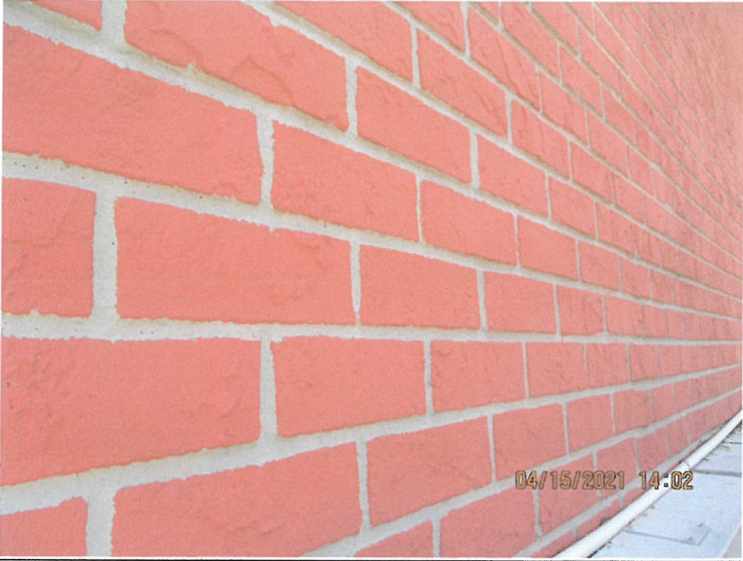
Building 1785-Example photo of brick façade with existing two-tone paint finish
