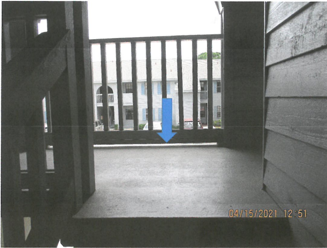
Building 1705-Example photo of proper drainage opening at bottom horizontal railing
