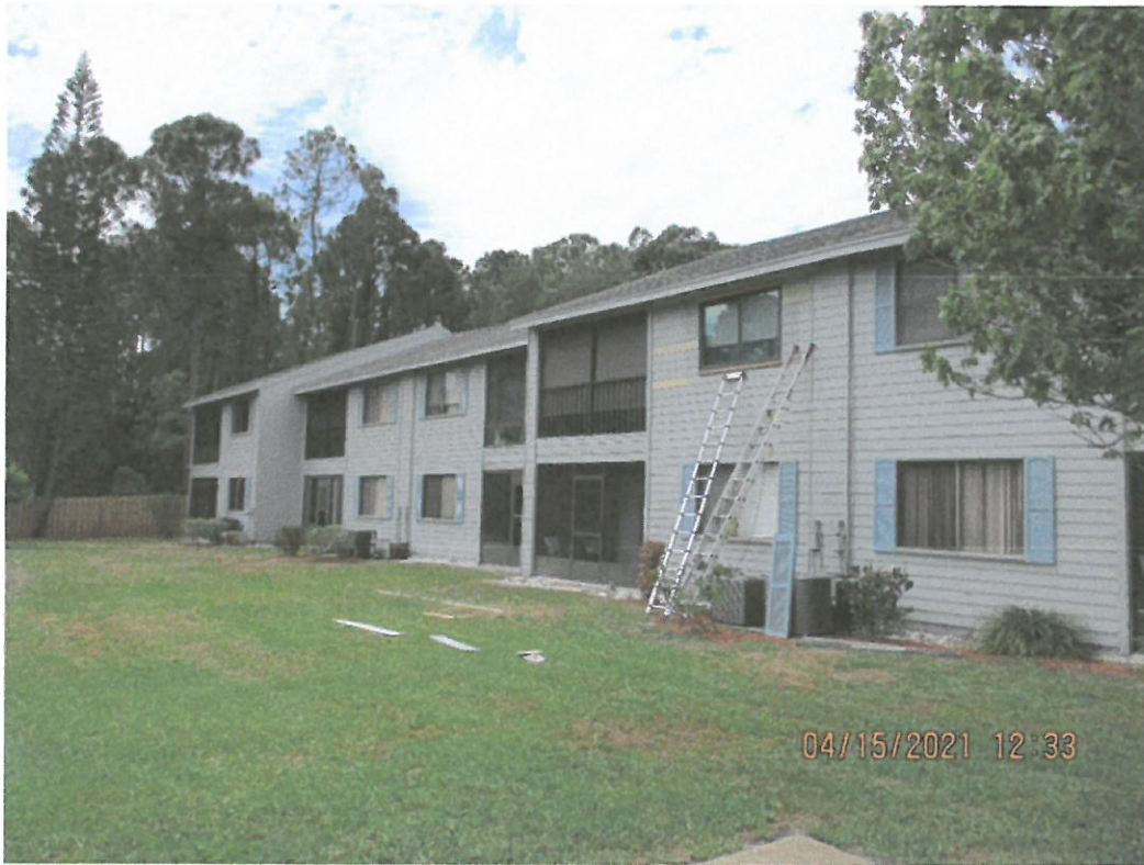
Building 1685-Example photo of siding repairs in process
