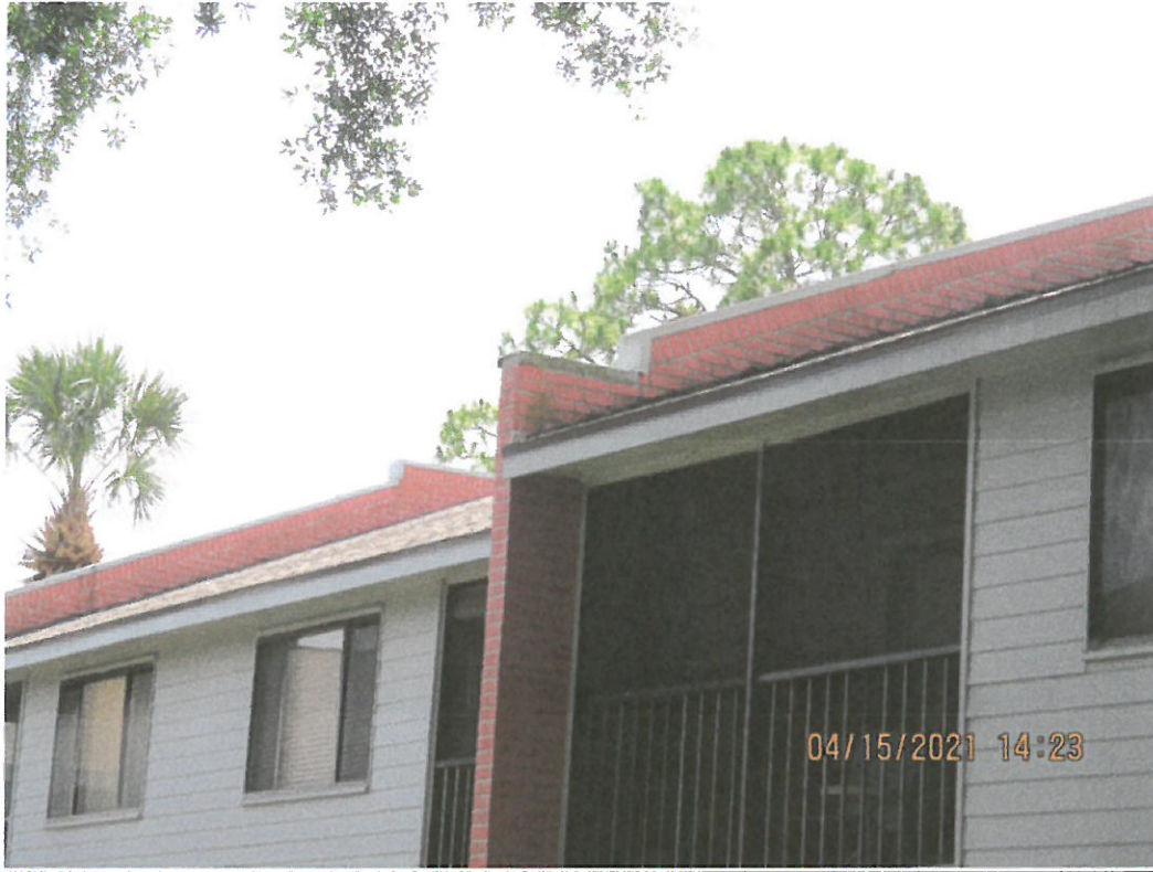
Building 1745-Example photo of brick façade stucco fire walls
