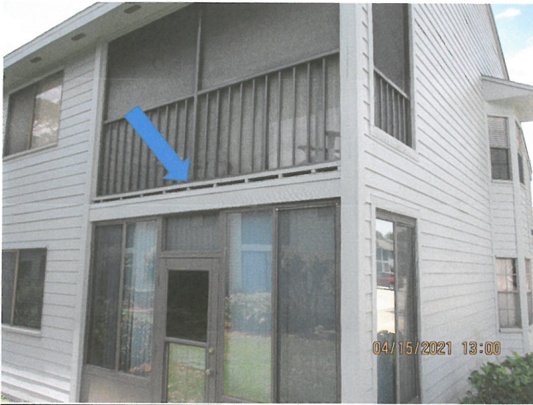
Building 1735-Example photo of proper balcony drainage from above
