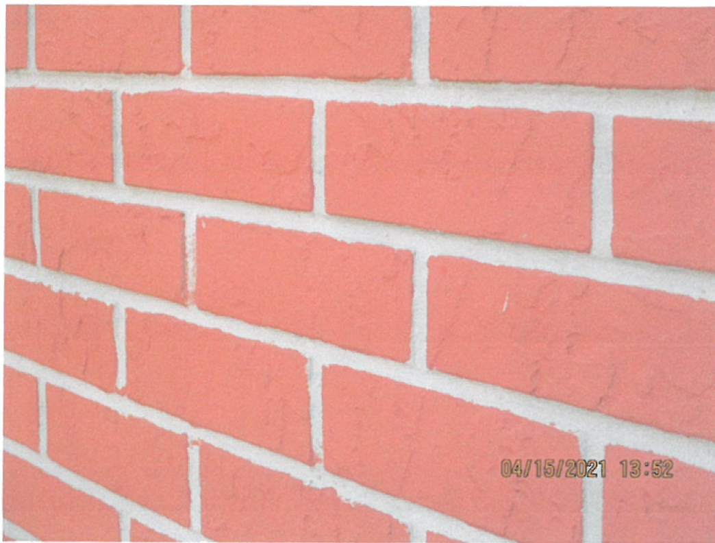
Building 1795-Example photo of brick façade with existing two-tone paint finish
