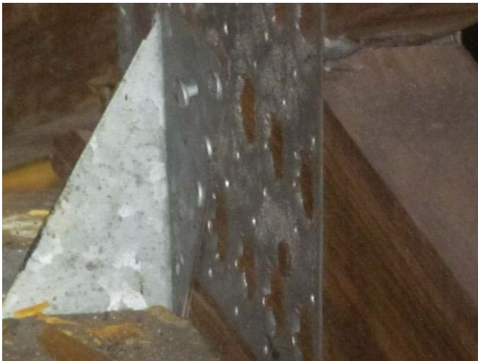
Clips - with minimum three nails
