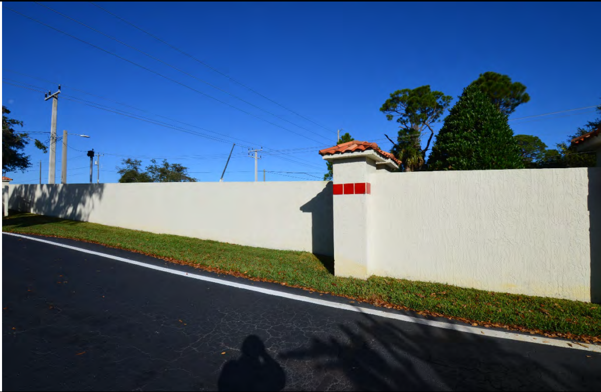
VIEW OF PERIMETER WALL
