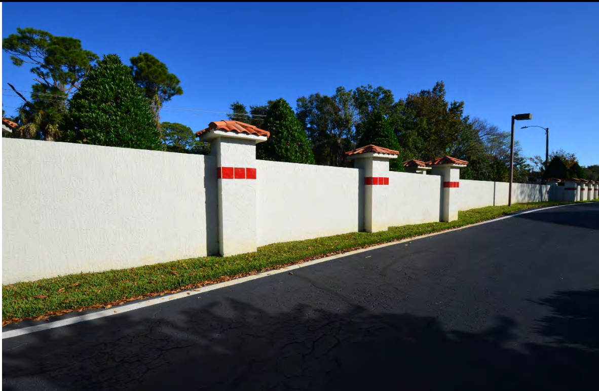
VIEW OF PERIMETER WALL
