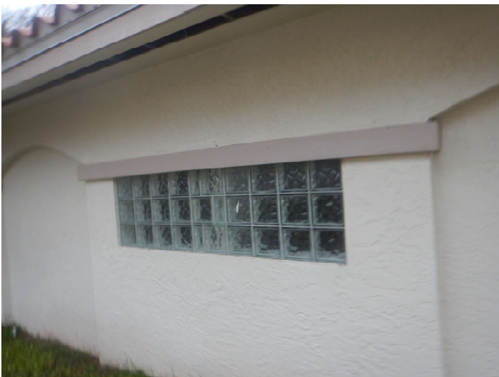
Glass block not required to be protected
