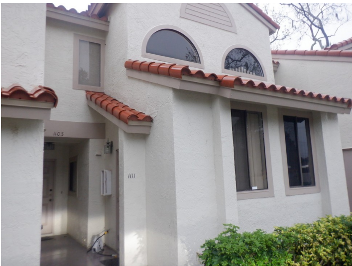
No openings protected
